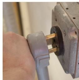
12. Plug the kiln back in and fire away! Monitor the kiln for the first few minutes to ensure the temperature is rising and if not, your thermocouple is installed in reverse.
