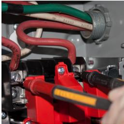
3. Open the cover of the control box and look for the two wires coming from your main breaker box. They will be secured into a metal block with set screws. Care-
