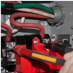
5. Carefully put one probe onto each of the screws making sure not to touch anything with the probe except screws. Take a note of the voltage. This is your
