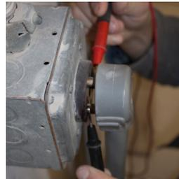
5. Carefully put one probe onto each of the flat blades making sure not to touch anything with the probe except the flat metal blade.
