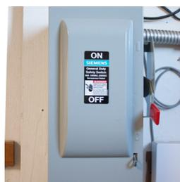
1. Push the control arm to the "Off" position (almost always down). The red handle is the control arm in this image. Open the cover of the shutoff box.
